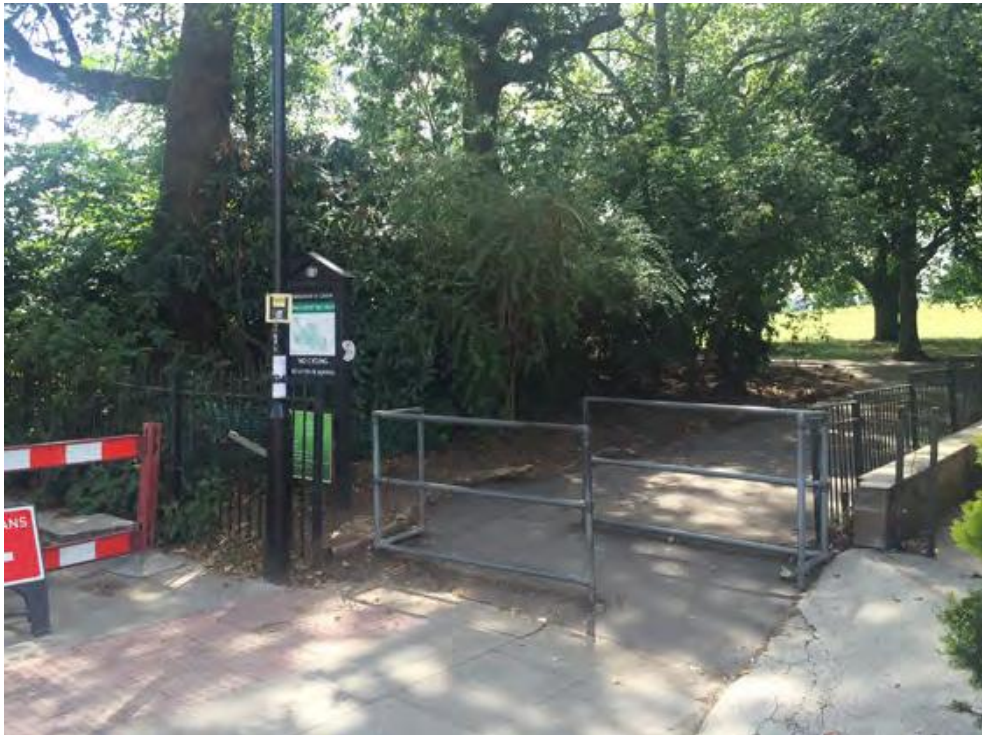
Figure 2 – Remove galvanised rails and replace with wooden posts. (Note 3, appendix 3 - proposed layout).
